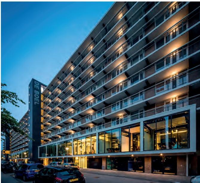
Apartment building de boel - Amsterdam - Netherlands
