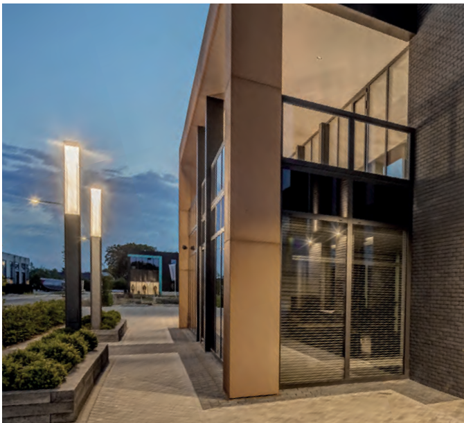
Robri - Wekerom - Netherlands
