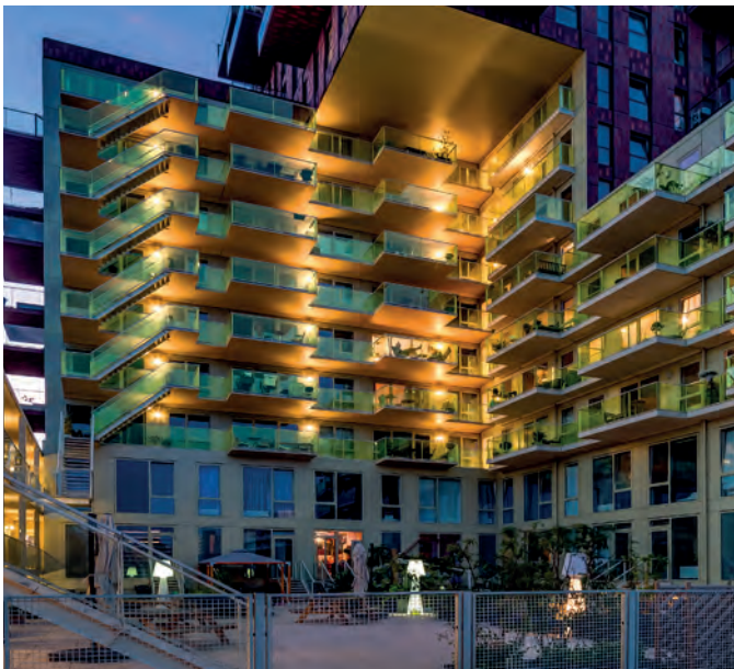
Residential Tower De Verkenner - Utrecht - Netherlands
