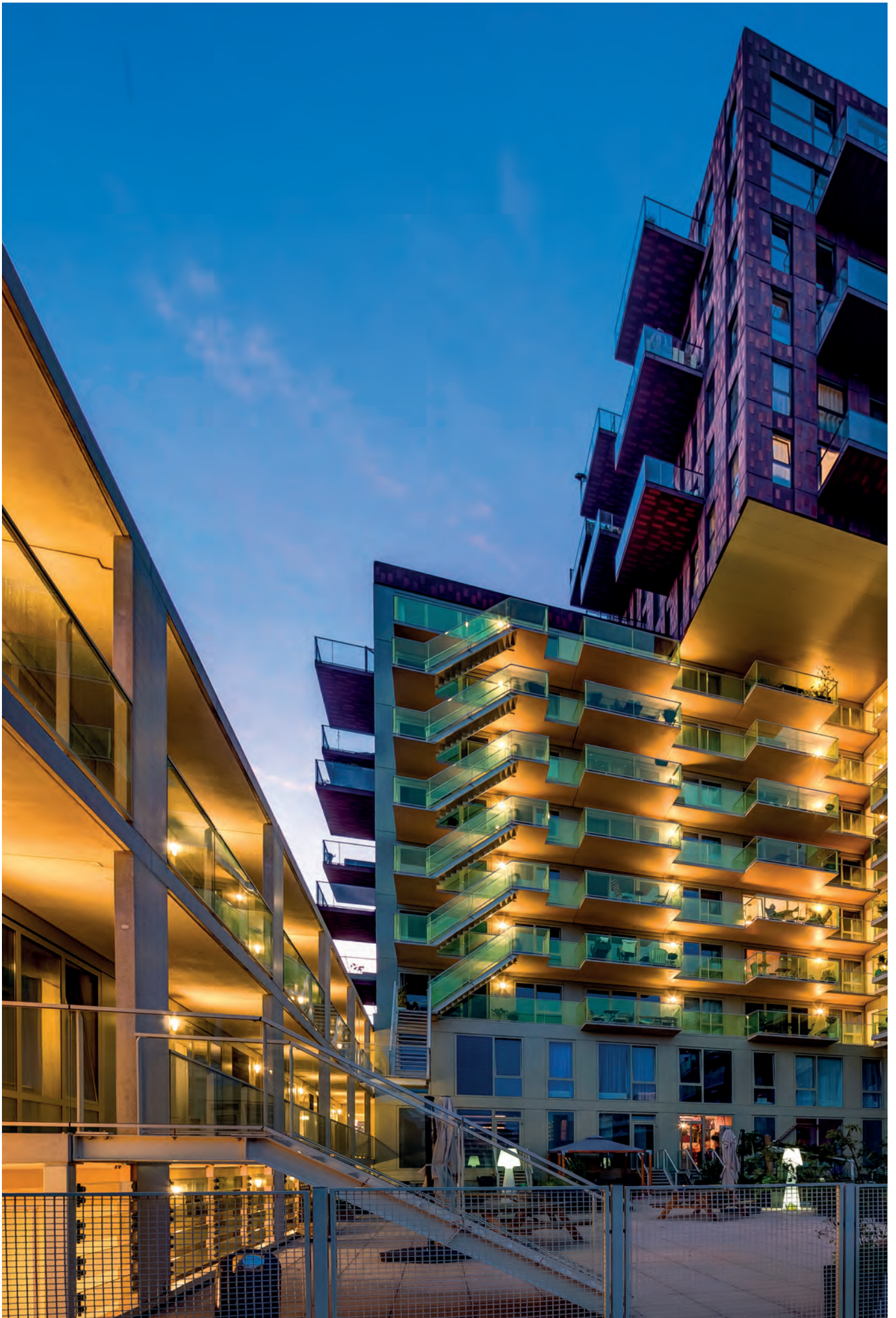
Residential Tower De Verkenner - Utrecht - Netherlands
