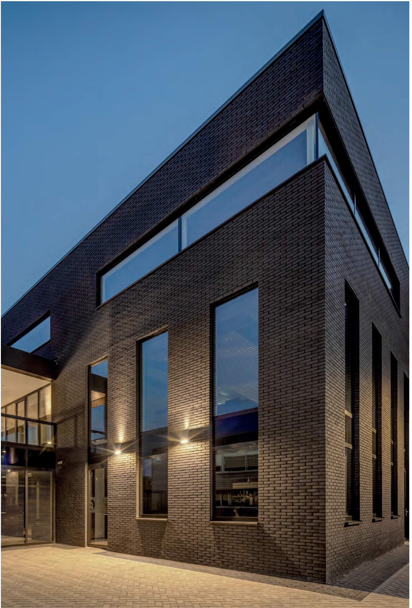
New Building Electrical Wholesaler Robri - Wekerom - Netherlands
